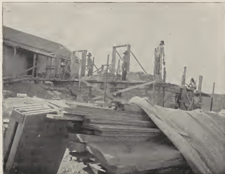
HOPIS AT WORK ON BUILDING AT SUNLIGHT MISSION.
